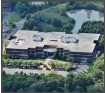
EAGLE ROCK EXECUTIVE OFFICE IV 120 EAGLE ROCK AVENUE EAST HANOVER, NEW JERSEY 177,820 SF ACQUIRED 12/17/14
